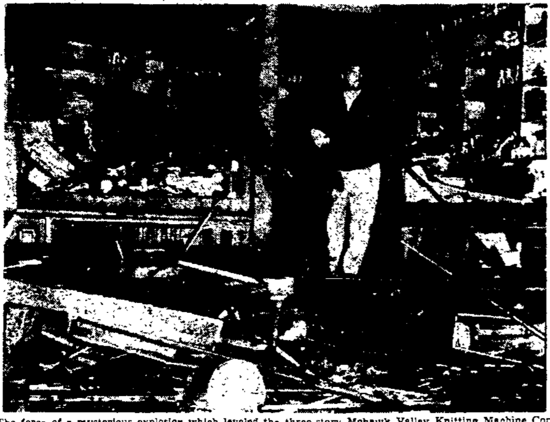
The force of a mysterious explosion which leveled the three-story Mohawk Valley Knitting Machine Corporation in Toledo, Saturday demolished the front of this grocery store, operated by Joseph Panetta. Twelve persons were injured in the blast. (Men unidentified. (AP Wirephoto).
