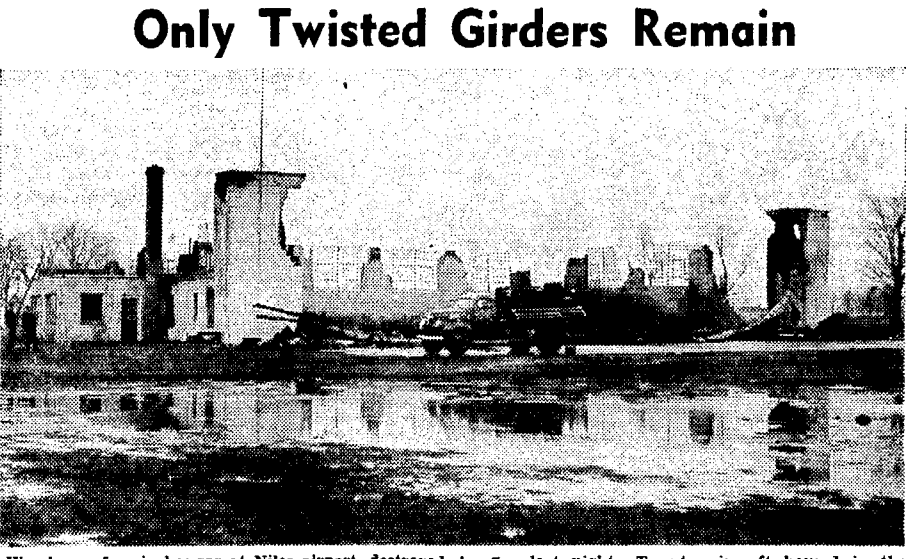
Wreckage of main hangar at Niles airport, destroyed by fire last night. Twenty aircraft housed in the hangar also burned.
