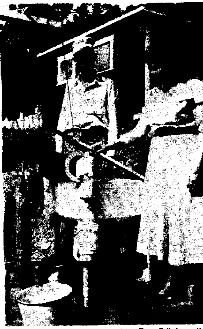
Wash day's a lark to Mrs. Ezra Templeton, Upper Falls housewife, since her menfolk hitched up a 25-year-old Maytag washer to draw water from her new, 125-foot-deep well. Her husband watches her operate the curious contraption.
