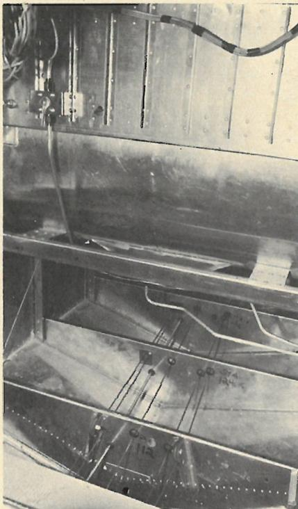
Teal's interior aft of cockpit details the fine workmanship. Fuel tank and spar are clearly shown. Un-chromated metal interior would soon corrode in salt water operations but production aircraft will be treated and protected in these vital areas.
